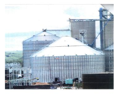
Construction on Ag Valley's Edison facility was completed on November 1, 2007, and the Titan model CB50 was placed into service. Final payment on the construction project was made by Ag Valley to Heartland on November 30. The Titan model CB50 was full of grain when it collapsed without warning almost 10 years later, on August 6, 2017.
